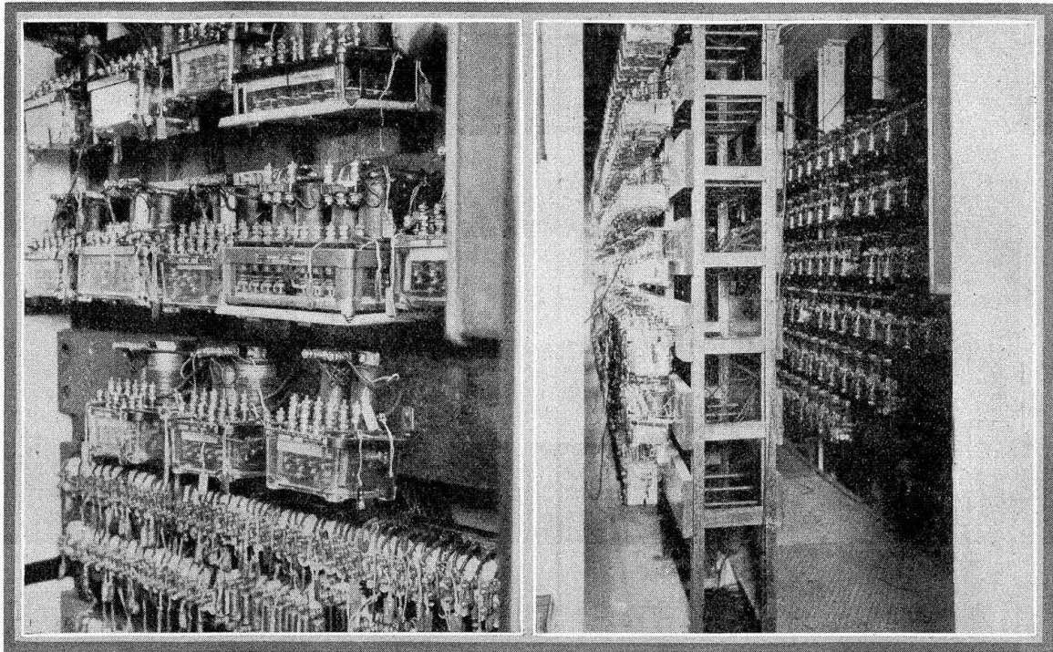
Interior of concrete relay house
